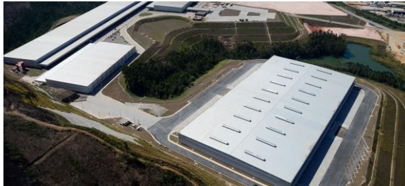
Distribution Park Cajamar
