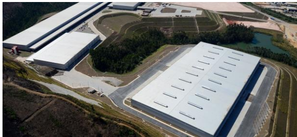
Distribution Park Cajamar
